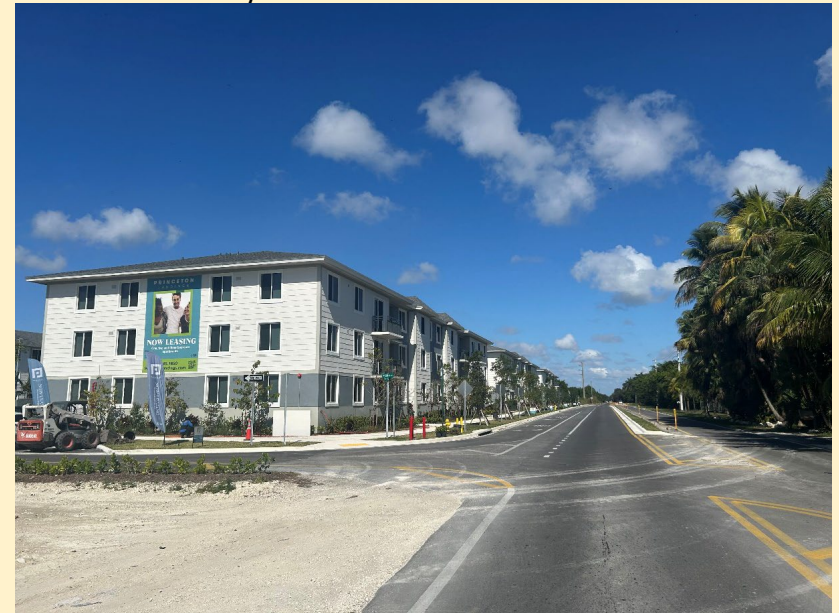
Princeton Landings development adjacent to application site, viewed from 127 th Avenue.
